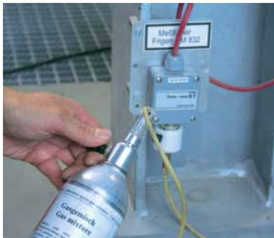
Figure 5: The function of a gas probe at ground level is checked by means of a test gas.
