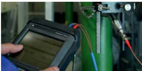
Figure 4: One of the ultrasonic probes, which transmits the flow-through data to the mobile measuring device.
